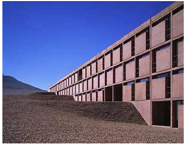
Chile: Hotel and Information Centre for the European Southern Observatory at Cerro Paranal Site-mixed concrete, pigmented with Bayferrox® 600 N
