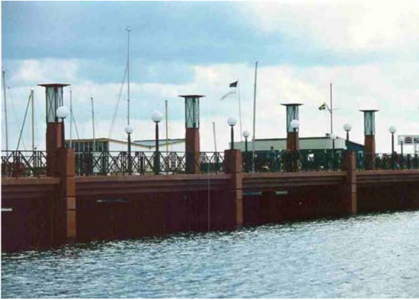
Sweden: Bridge: Kvick Bron, Helsingborg Site-mixed concrete, pigmented with Bayferrox® 130
