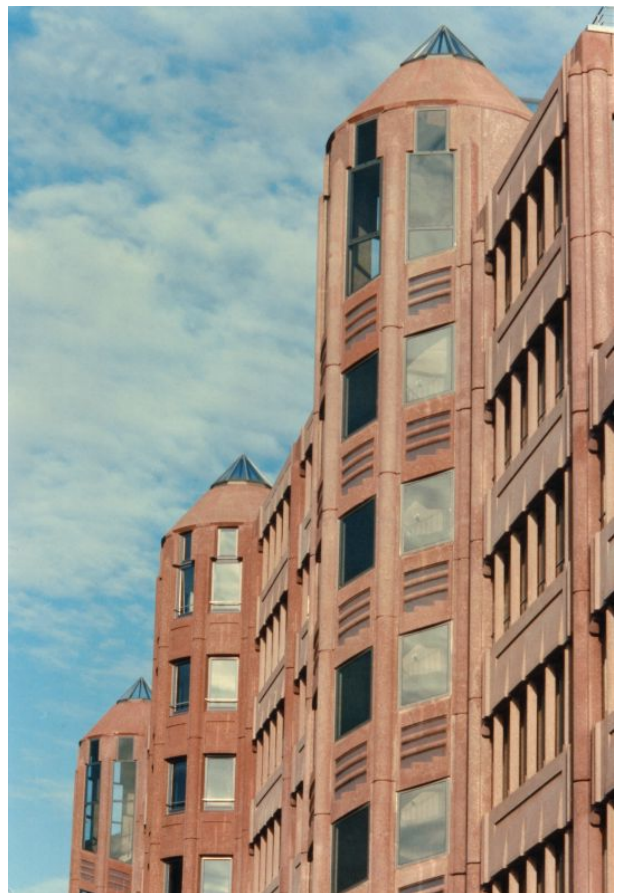
Germany: Administration Building of Zueblin AG, Stuttgart, Precast Elements, pigmented with Bayferrox® 110
