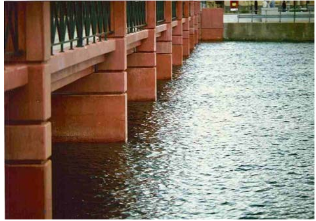
Pigment concentration: 6 % Built: 1995 – 1996 Architect: Nilsson & Rahmquist, Helsingborg Building company: Ballast Syd, Helsingborg
