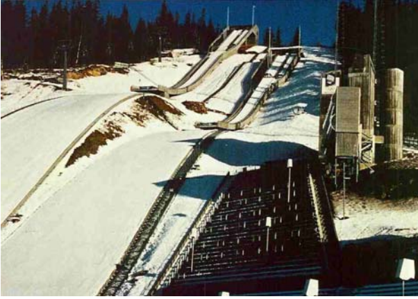
Norway: Olympic arena, Lillehammer (Lysgaard skijump); Site-mixed concrete, pigmented with Bayferrox® 318
